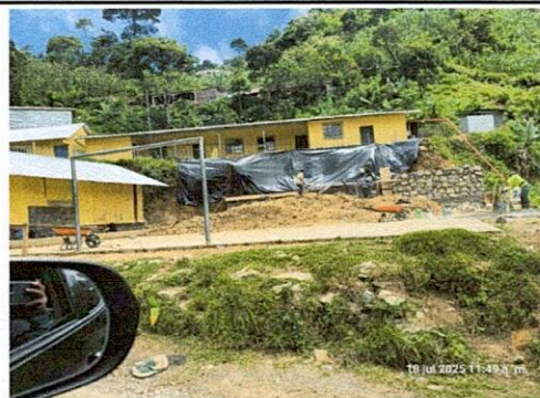
Foto 6: Vista general frontal
